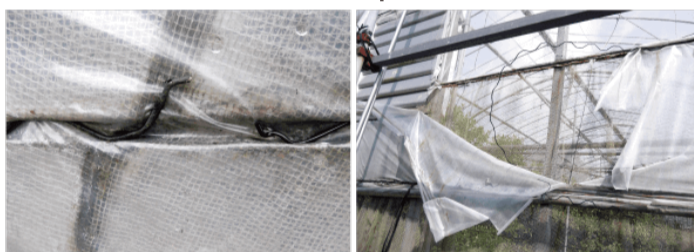
Difficulty cutting both ends (easy to lift up and scratch the plastic film)
